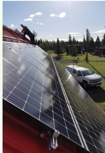
Option 7C: Standing seam metal roof clamps
