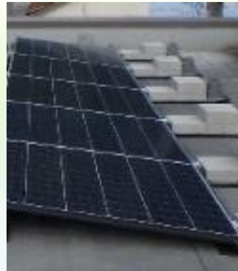
Option 7D: Ballasted systems on flat roofs
