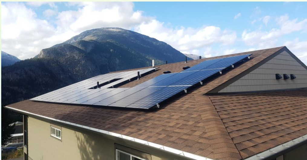
“Solar Ready” South Roof Peppered with Vents
