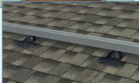
Option 7A: Flashed anchors secured into roof sub-structure
