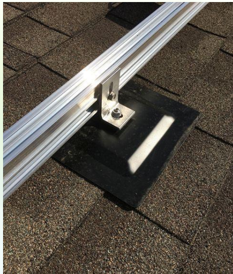
Option 7B: Flashed anchors secured into roof decking
