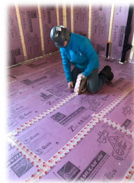
RADON BARRIER SYSTEM
