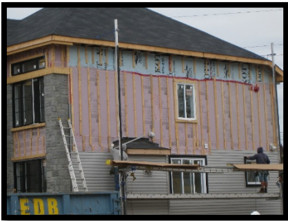
Attachment of Cladding Through Continuous Insulation
