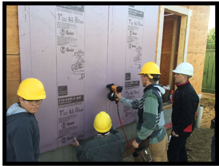
Attachment of Cladding Through Continuous Insulation
