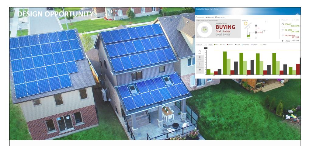
Push ridgeline forward and drop pitch to contain all needed panels Reduce array to a maximum of 32 panels – 8.5 KW
